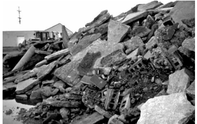
Mitchell stockpiles both salvage asphalt and concrete and then crushes and blends both materials for use as base in new construction.
