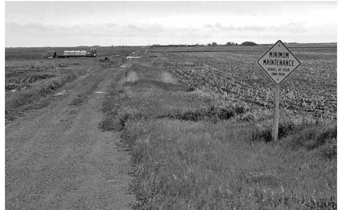
This is a good example of a road that serves only as a field access and is designated and signed properly as minimum maintenance.
